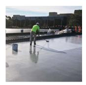
To ensure that all sections of the roof – including the areas under and around cooling and other equipment – were fully waterproofed, the Coniroof 2160 waterproofing application was completed as a three-stage process, carried out before, during and after the air-conditioning and other equipment was installed.
